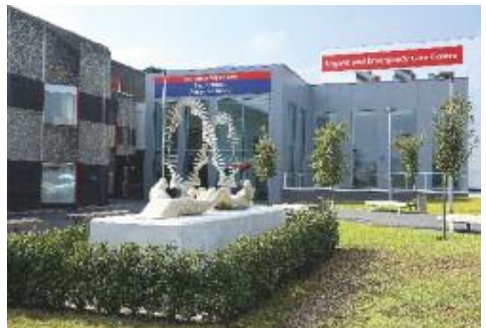
Nucleus and Heart/Lung theatres at Wolverhampton's New Cross Hospital are supported by the TissueSAFE system.
